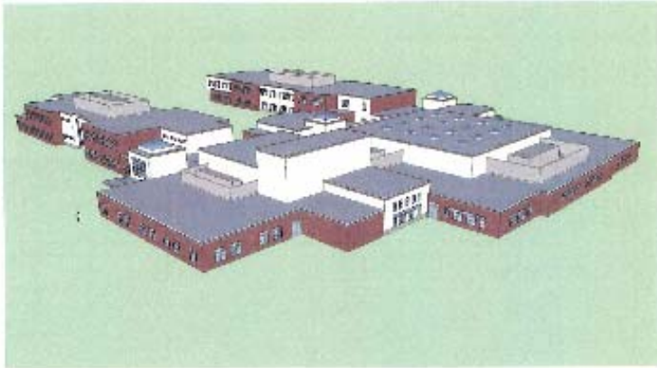
SOUTH EAST AERIAL
