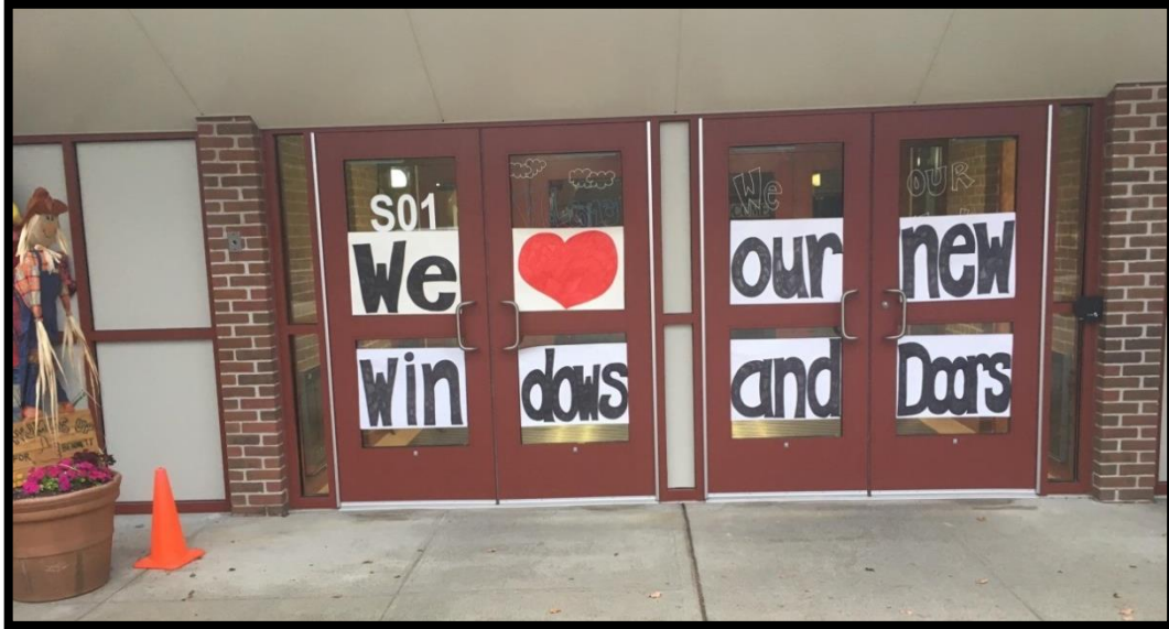
The photo above was received from the Edmund Hatch Bennett School in Taunton, a 2015 ARP Invitation. The project was completed in September 2017, which included repairs to the Roof, Windows, and Doors.
