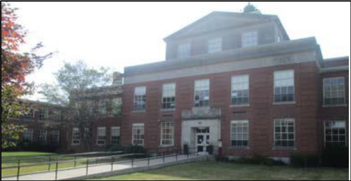
The photos above and below depict Wellesley Middle School, a 2014 ARP invitation, before and after a window/door replacement project, which was completed in September 2016. The project is a candidate for Final Audit Approval at the August 2018 Board of Directors Meeting.
