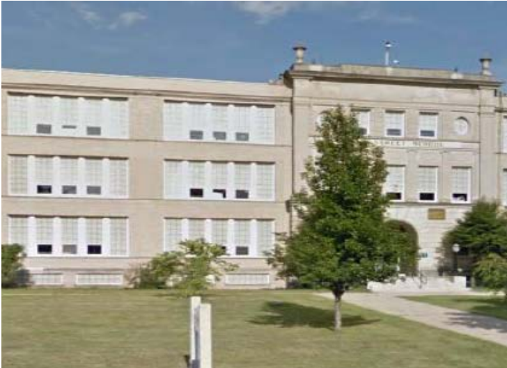
The photos above and below depict the before and after of the Elm Street School in Gardner, serving 554 students. The project replaced the windows, doors, and boilers and will extend the useful life of the 93-year-old building. The project reached Substantial Completion in November 2016 and is being brought to the April 2019 Board of Directors meeting for Final Audit Approval.
