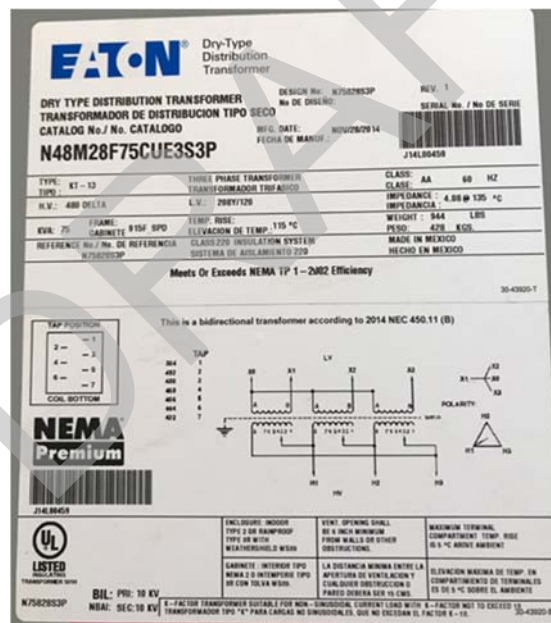
Figure 18. K-rated Transformer TC1A
