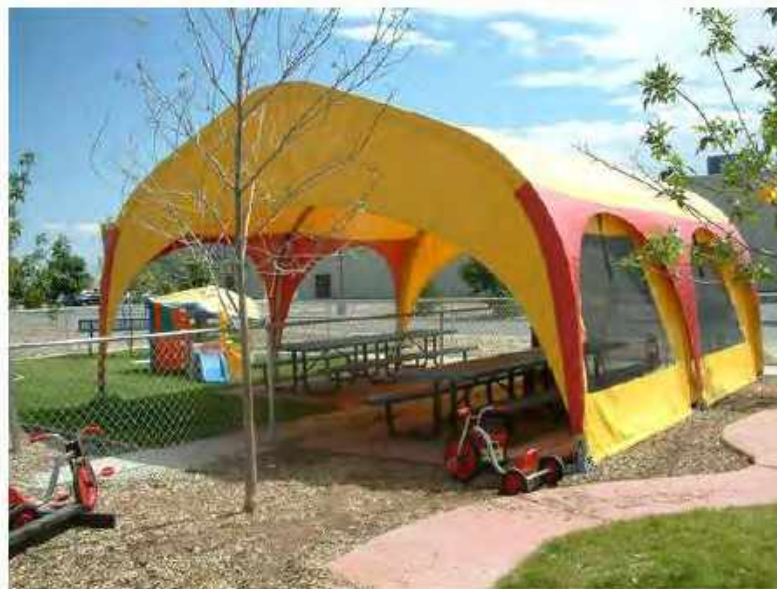
21' Wide x 20' Long Outdoor Classroom Structure For Additional Classroom Space
