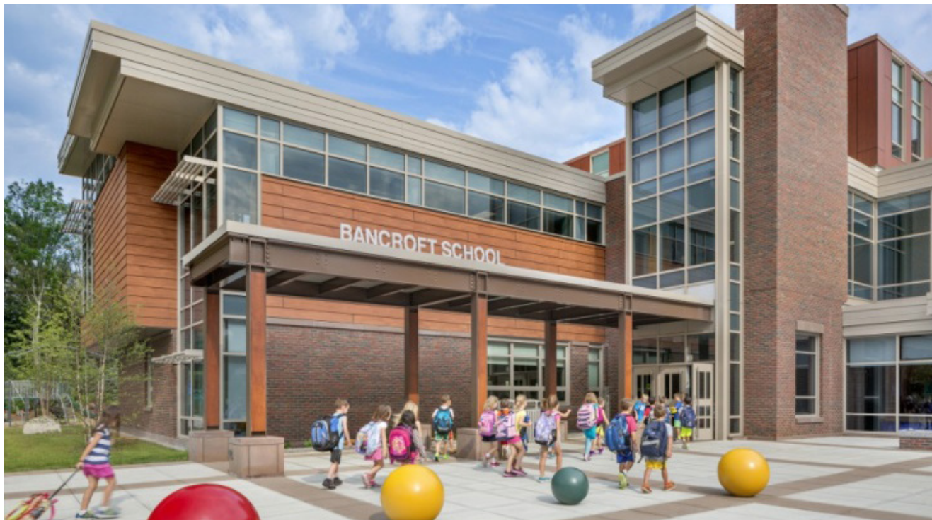
Bancroft Elementary School, Andover
