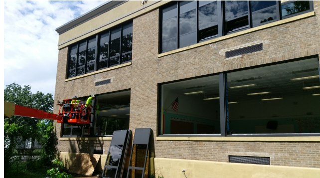
ARP Window Project at Barrett Russell School, Brockton
